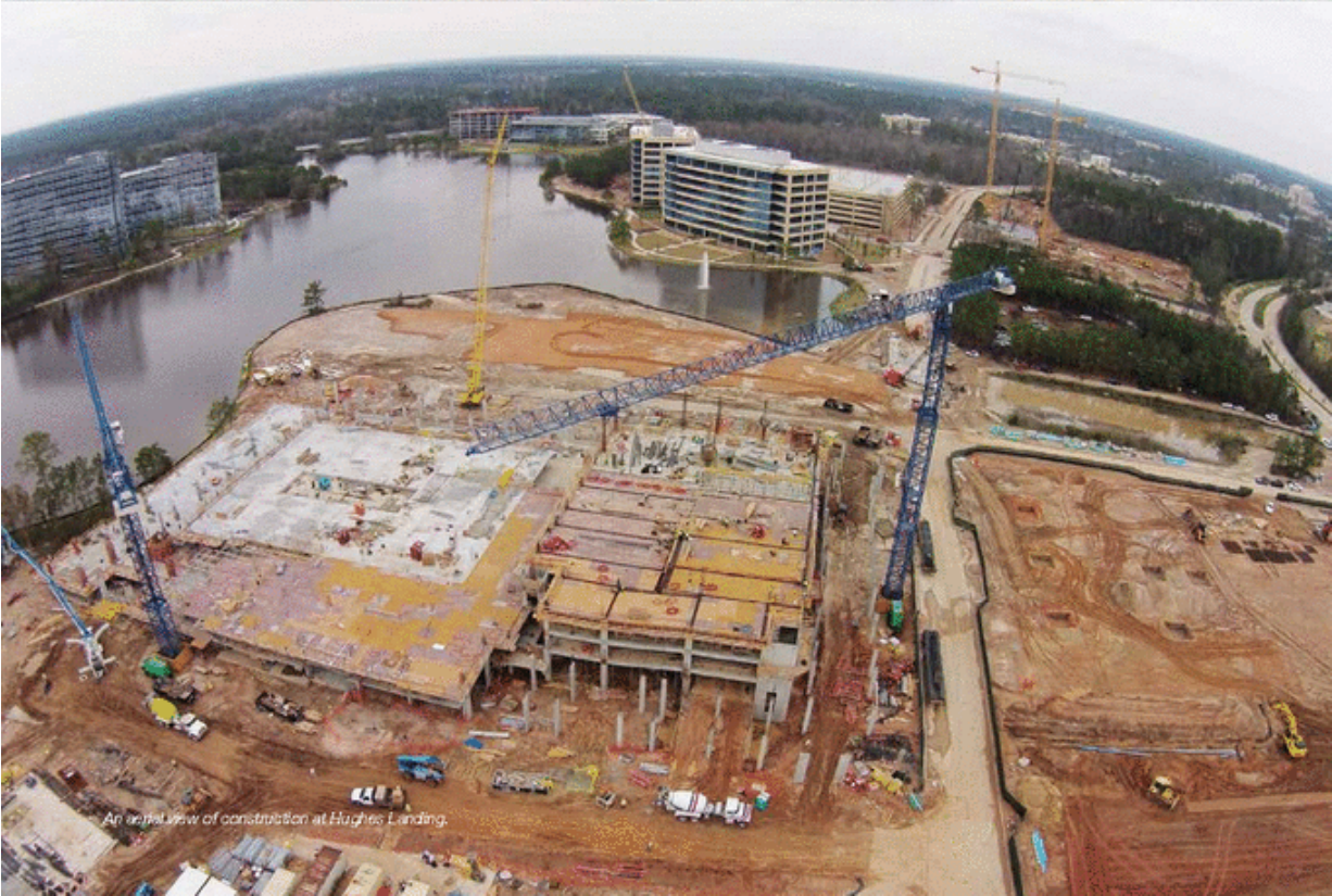
An aerial view of The Shops at Summerlin under construction.
