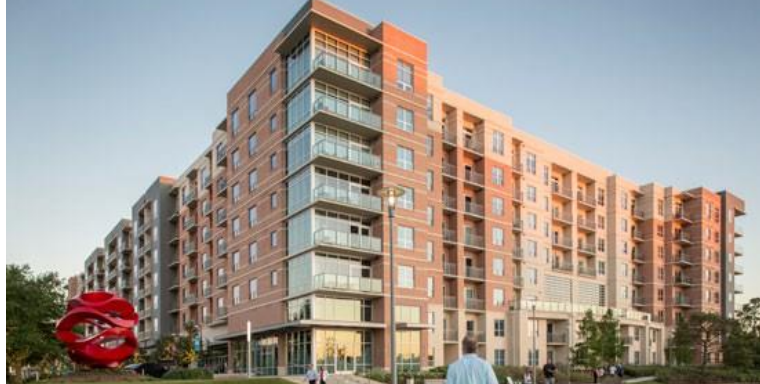
Built and operated by Howard Hughes
