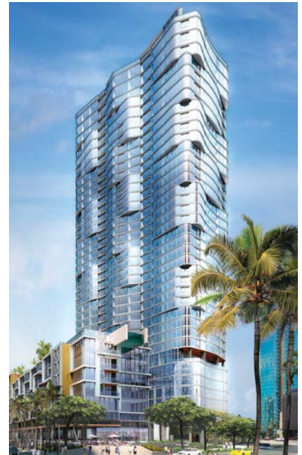
Anaha Tower—Part of our first phase, Anaha is the Hawaiian phrase for “reflection of light,” and describes the building’s brilliant, rolling glass façade, which evokes the rippling waves of the nearby Pacific Ocean.
