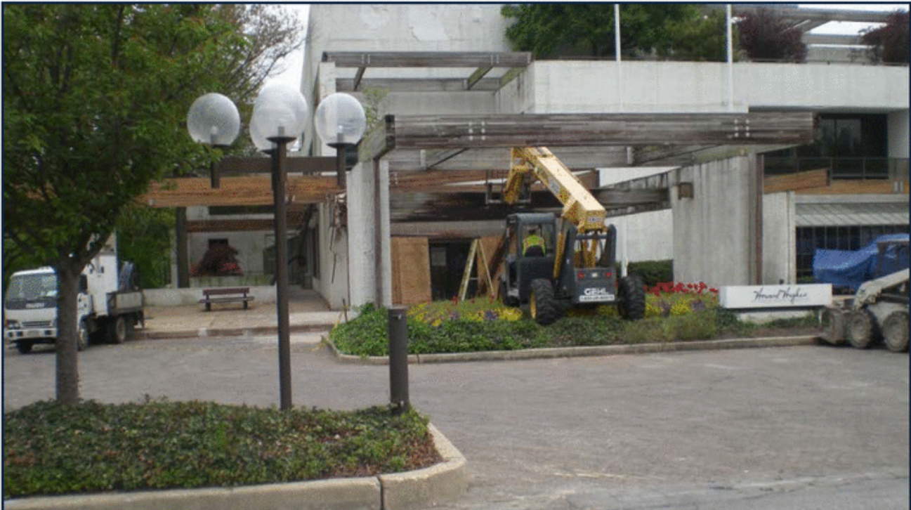
Breaking Ground on Redevelopment – May 2013
